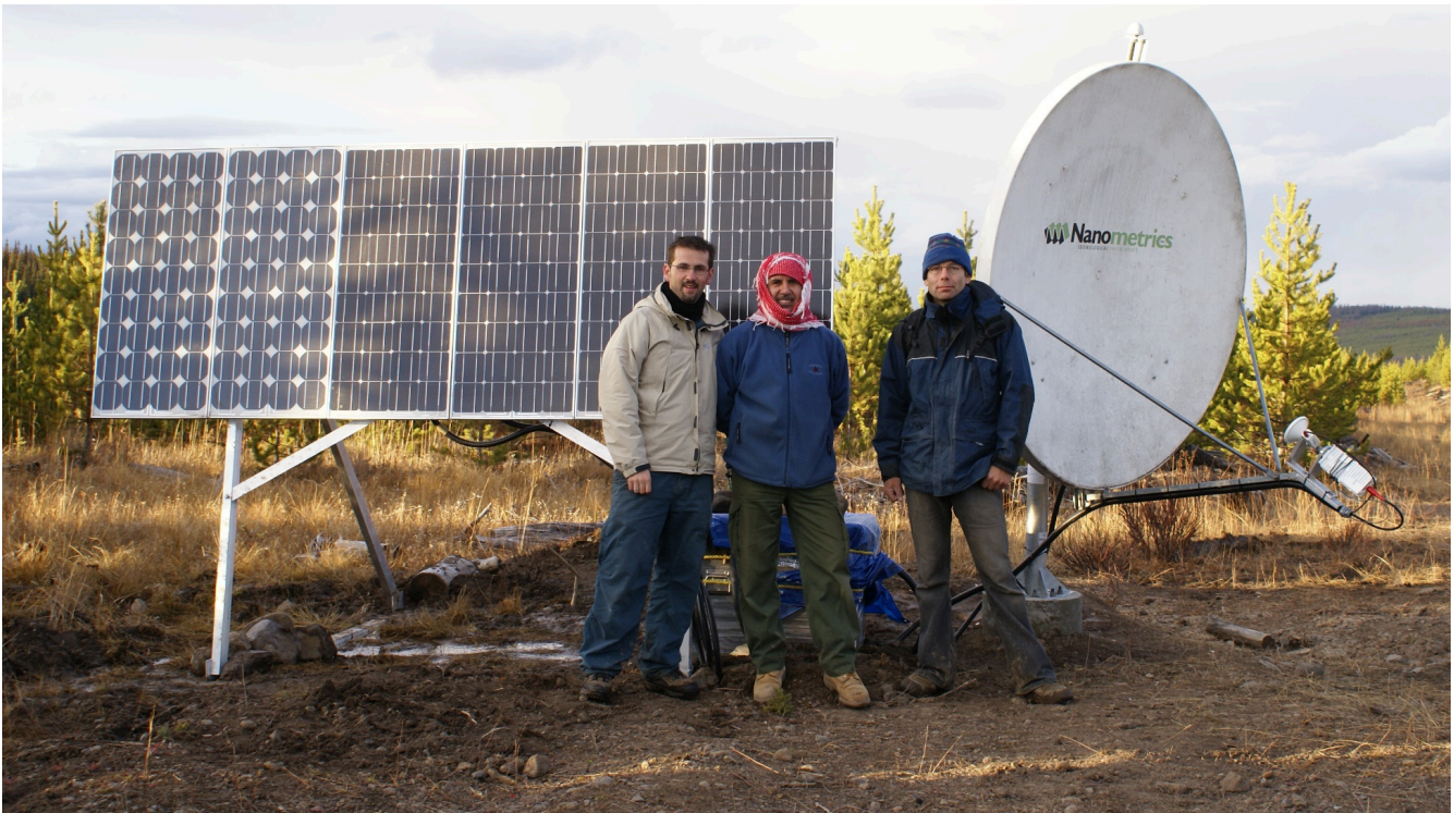
Figure 4.5.1 A seismometer and related power and communication equipment installed in 2007 in the vicinity of the Nazco Cone, British Columbia
