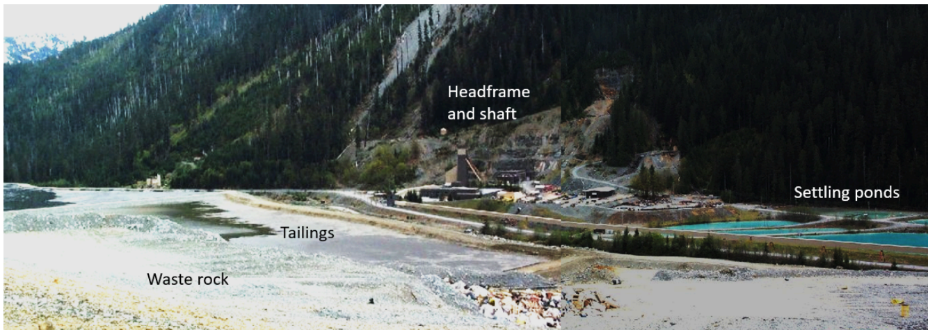
Figure 20.1.10 The tailings pond at the Myra Falls Mine on Vancouver Island. The dry rock in the middle of the image is waste rock. Myra Creek flows between the tailings pond and the headframe. The settling ponds (right) are used for processing water from the concentrator.
