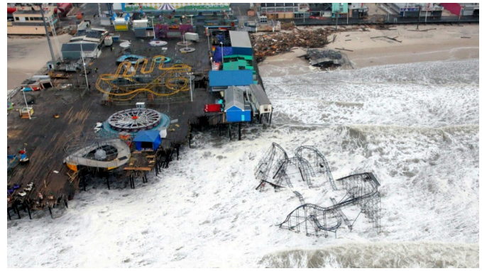
Figure 19.3.2 Damage to the Casino Pier, Seaside Heights, New Jersey, from Hurricane Sandy, November 2012.
