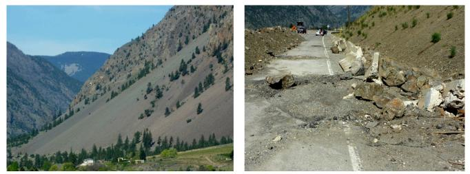
Figure 15.2.2 Left: A talus slope near Keremeos, B.C., formed by rock fall from the cliffs above. Right: The results of a rock fall onto a highway west of Keremeos in December 2014.
