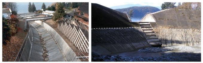
Figure 15.3.6 Two strategies for mitigating debris flows on the Sea-to-Sky Highway. Left: A concrete –lined channel on Alberta Creek allows debris to flow quickly through to the ocean. Right: A debris-flow catchment basin on Charles Creek. In 2010, a debris flow filled the basin to the level of the dotted white line.
