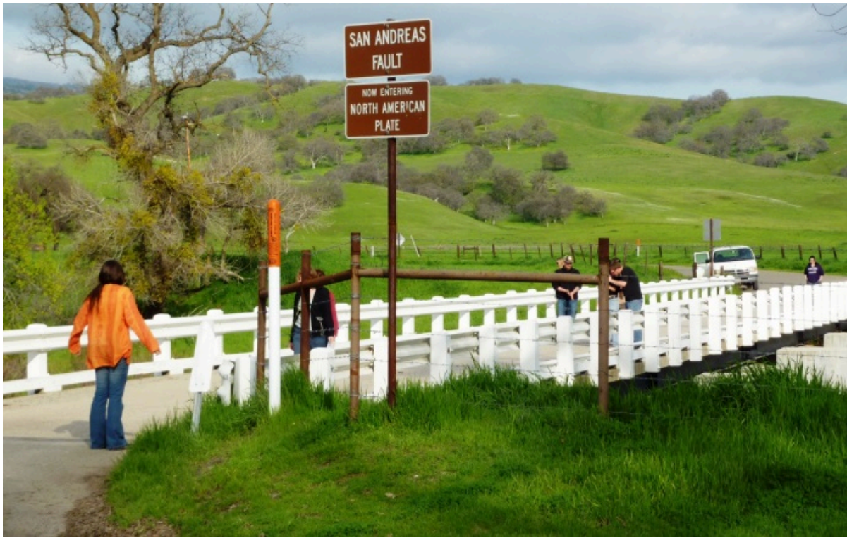
Figure 10.4.10 The San Andreas Fault at Parkfield in central California. The person with the orange shirt is standing on the Pacific Plate and the person at the far side of the bridge is on the North American Plate. The bridge is designed to accommodate motion on the fault by sliding on its foundation.
